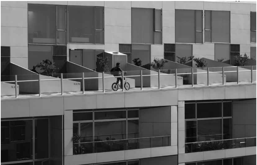
Fig. 1 - The 8-House: A pathway winding up along the facade makes it possible to walk or even bicycle to the top of the building.
